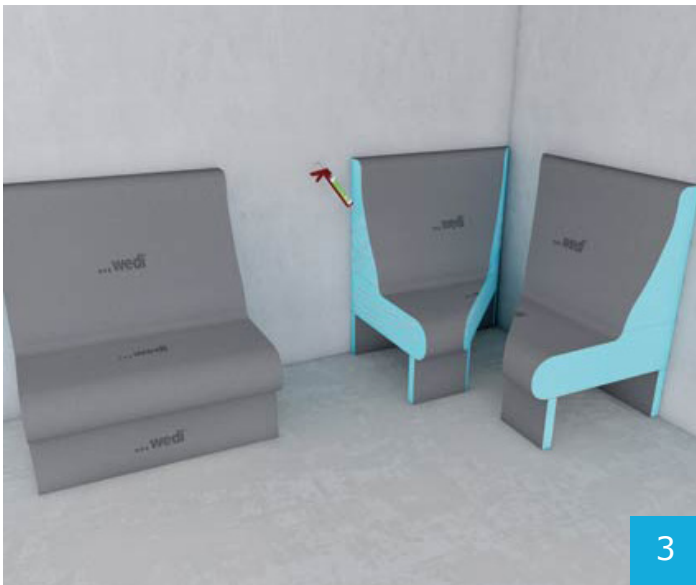
Connect the bench elements by using wedi 610 adhesive sealant...
