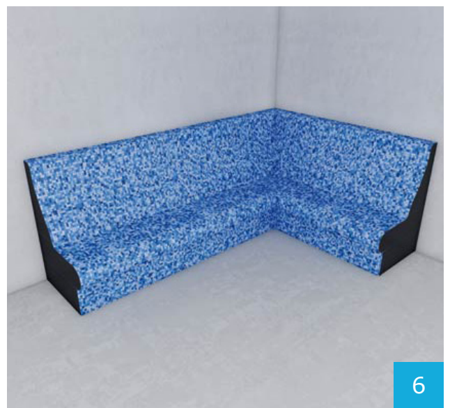
Then, the bench elements can be individually tiled.
